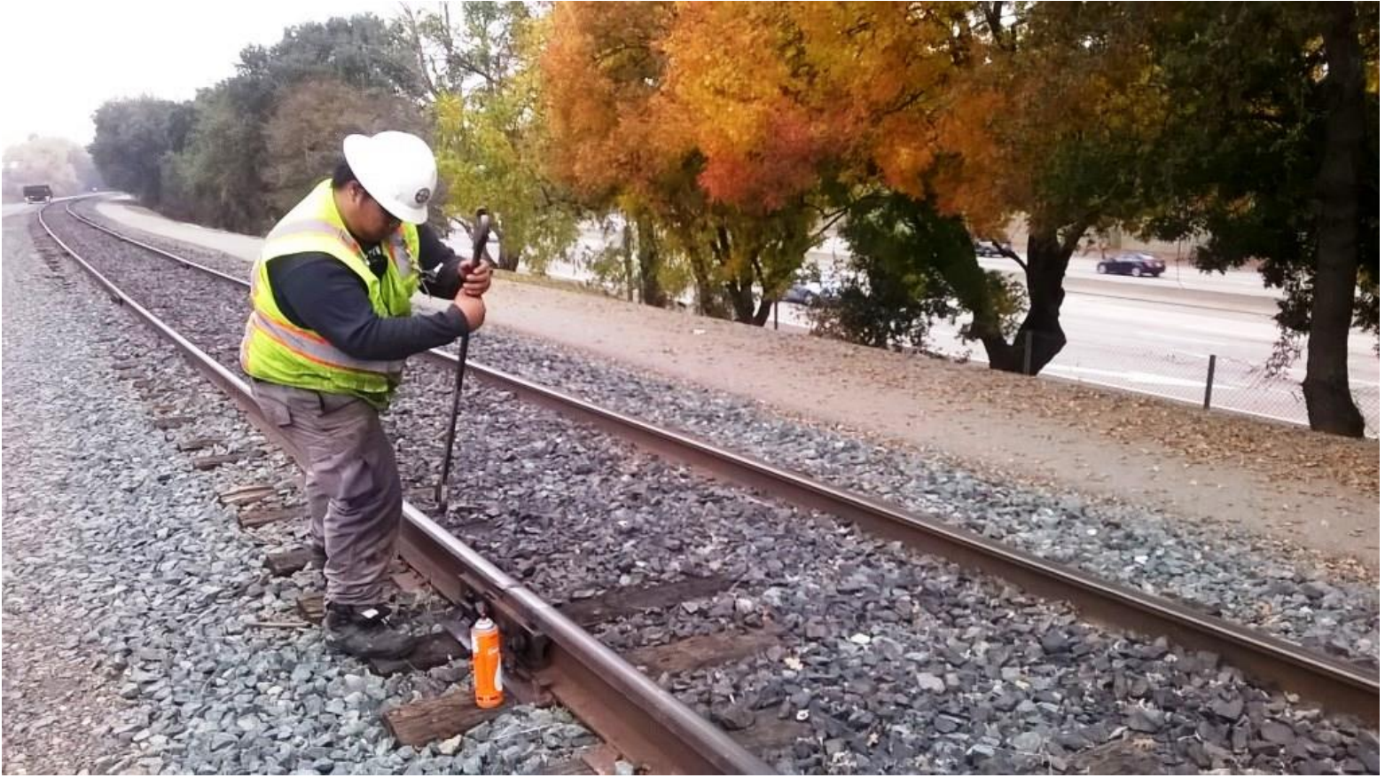
At Mile Post 2.4, Anthony tightens down the new bolt
