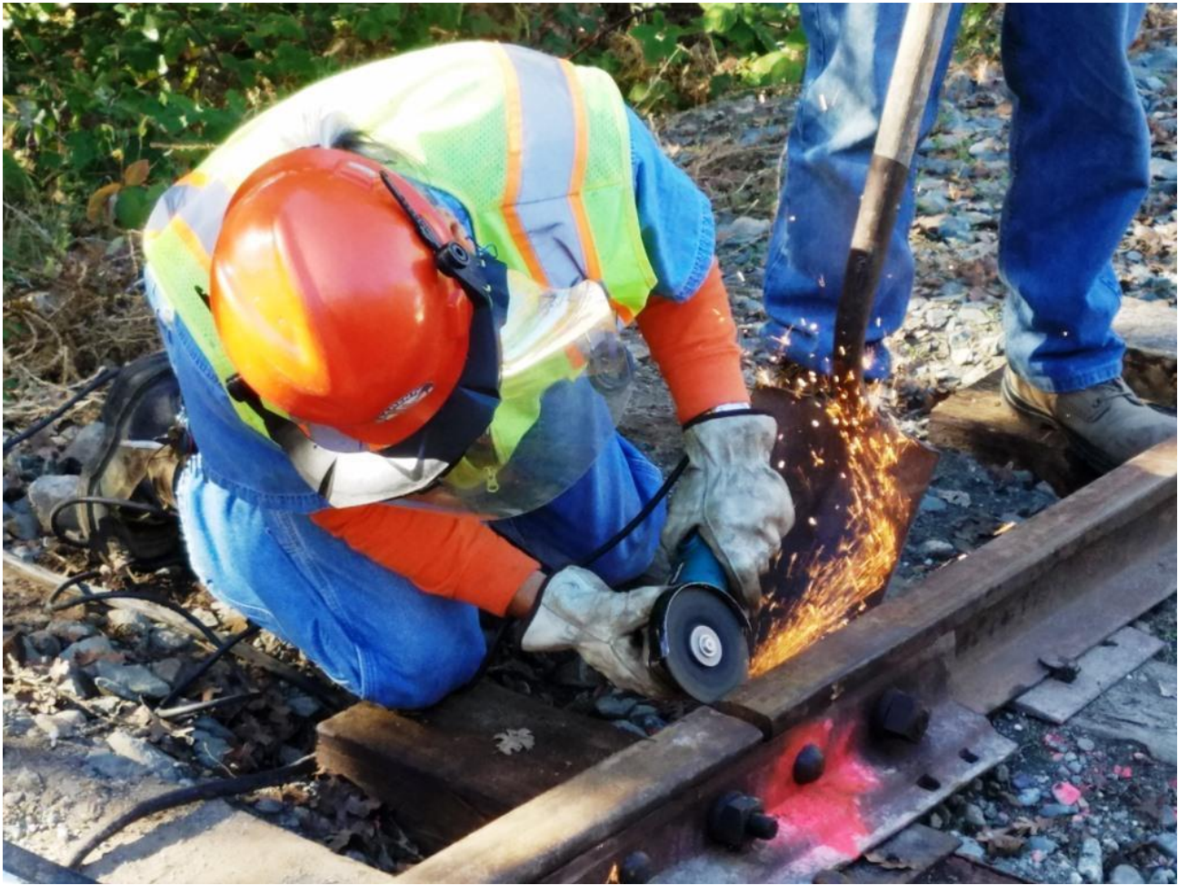
Ed grinds the old bond-wire welds off the rail
