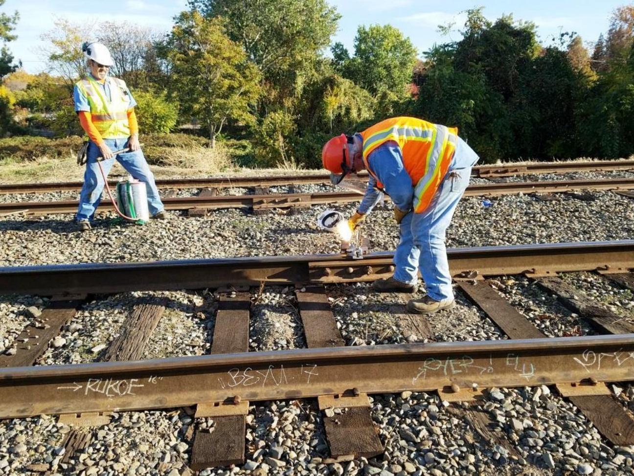
Joe ignites the thermite which will bond the wonky bond-wire to the rail at Clunie
